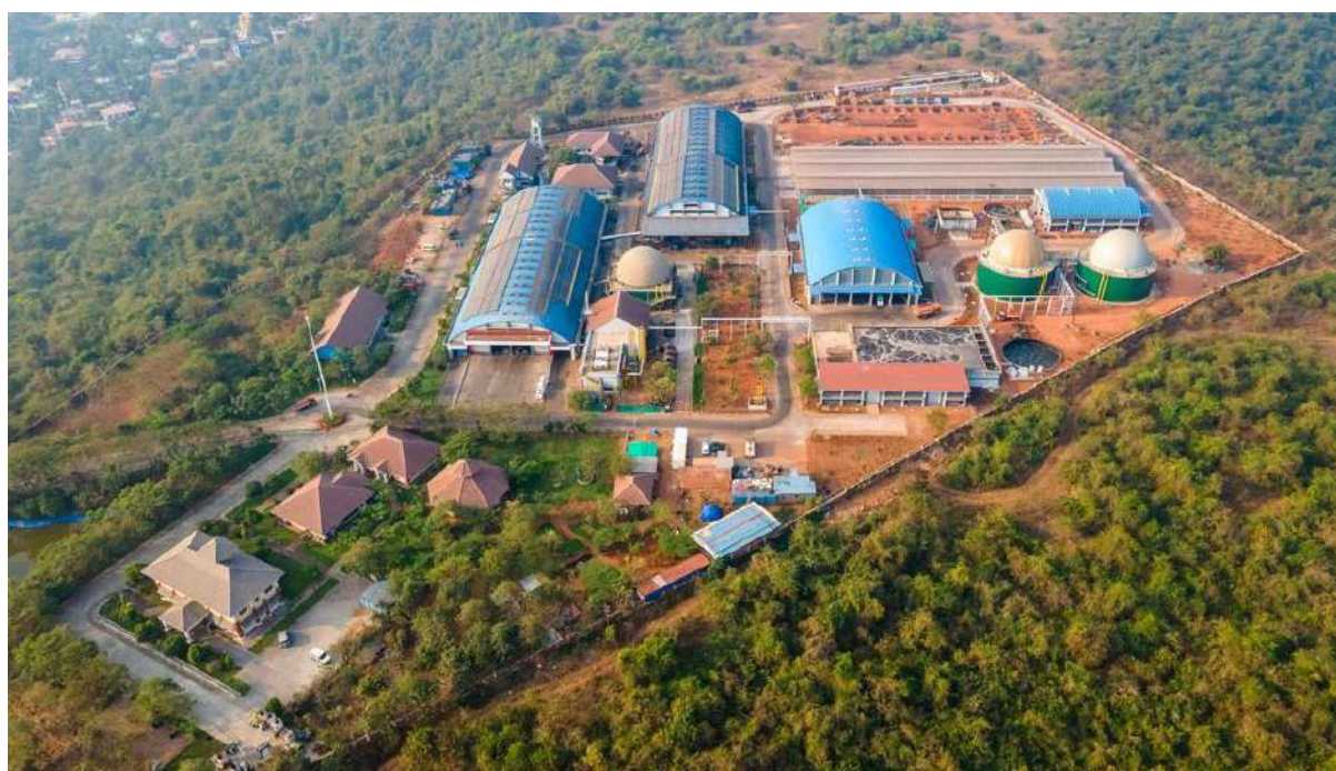
North Goa Plant
